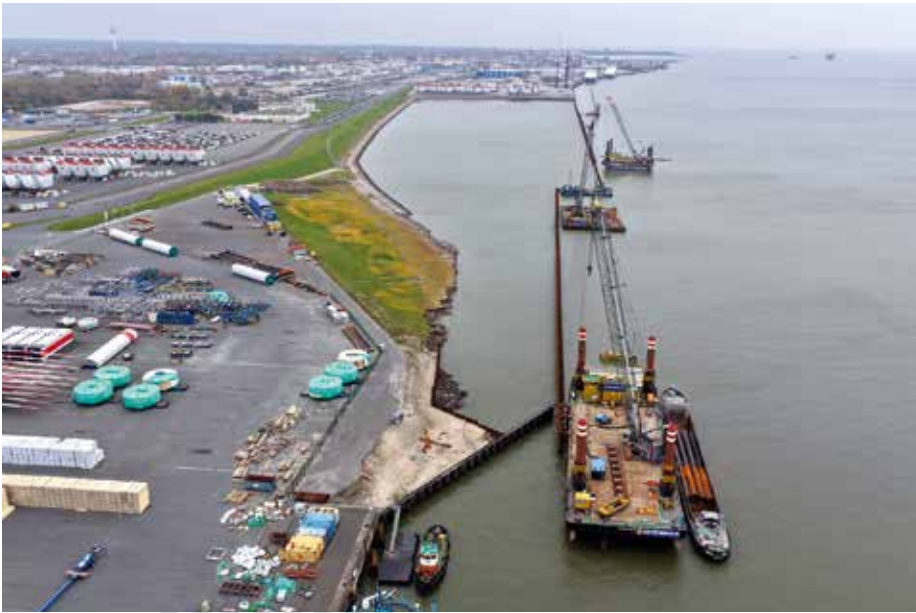
Three new heavy-lift berths will be built in Cuxhaven by 2028 as part of the offshore port’s expansion.
