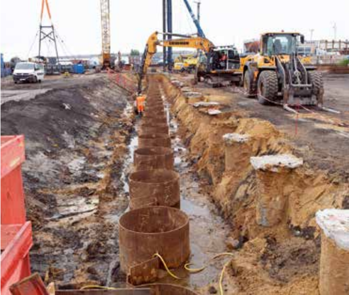
The redevelopment of the West Quay in Bremerhaven will create more space, both for building converter platforms for offshore wind energy and for manoeuvring large ships.
