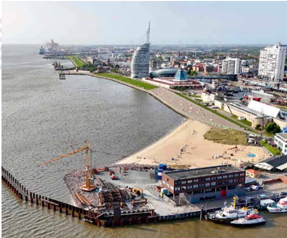
Construction of the new jetty in Bremerhaven is in full swing. The new structure will be 280 metres long and feature the historic lighthouse as its landmark.
