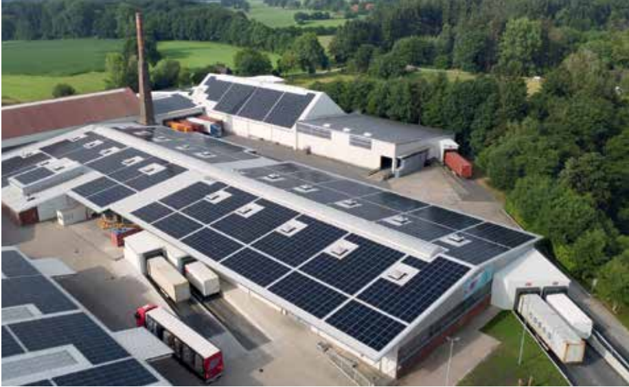
Thanks to a large five-megawatt photovoltaic system on the roofs, Albers Logistik's sustainable approach is also visible from above.
