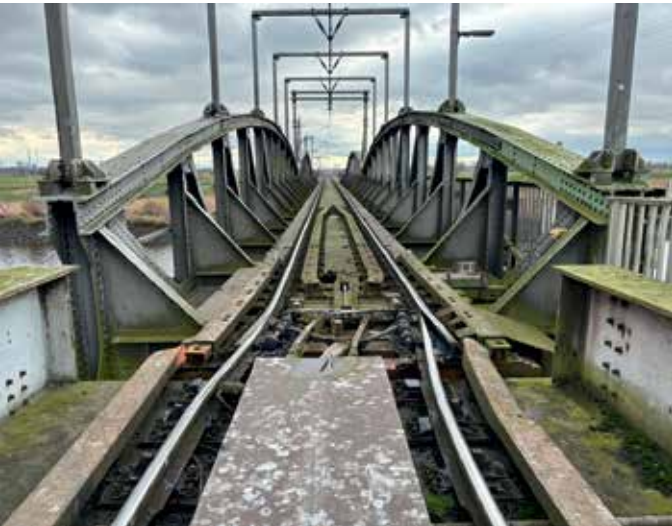
The ship accident severely damaged the bridge, the rotating structure, and the rail and overhead contact line system.
