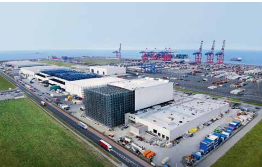
The high-bay storage system at NORDFROST Seaport Terminal in Wilhelmshaven was built in around 14 months and has been operating since November 2021.
