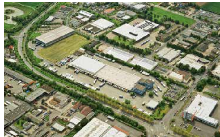
PHOTO: ZUFALL LOGISTICS GROUP; ZUFALL LOGISTICS GROUP/CHRISTIAN WOLTER
