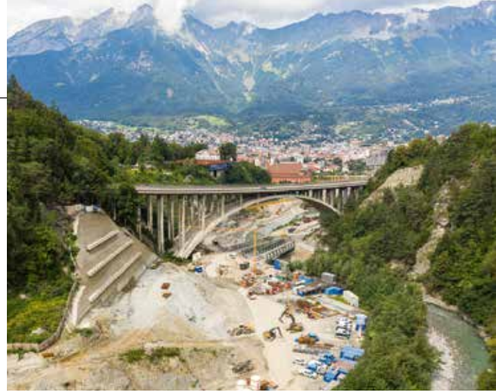
There's much to be done to complete the BBT – such as slope removal work here on the Bergisel to build the 'Silltal' pre-tunnel.
