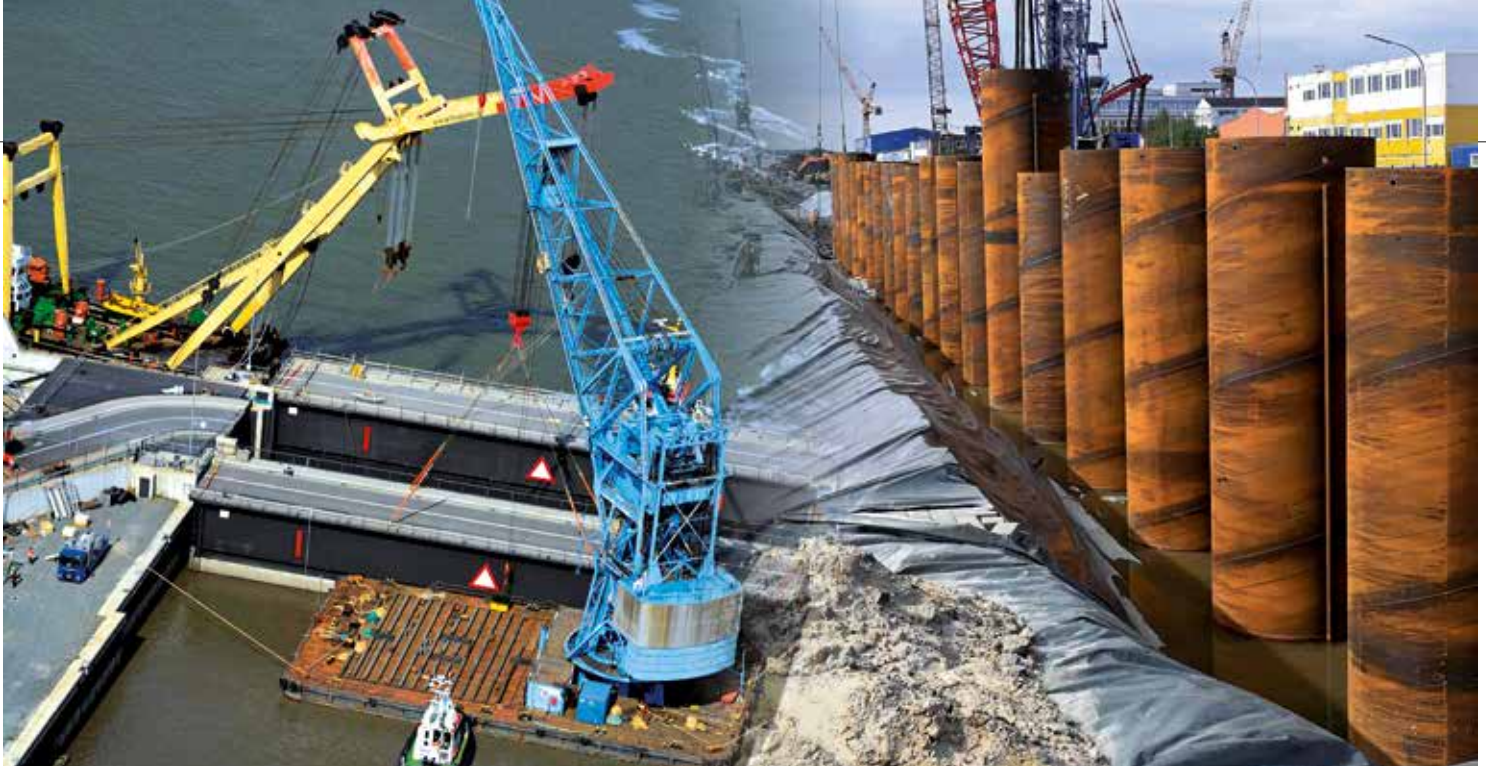
The Kaiserschleuse (l.) and Westkaje at the Kaiserhafen (r.) are just two examples of the many infrastructural measures in Bremerhaven.
