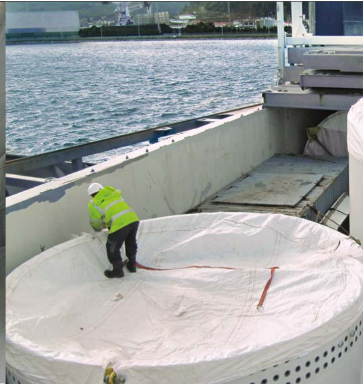
The base sections of the wind turbines are loaded on board by crane.
