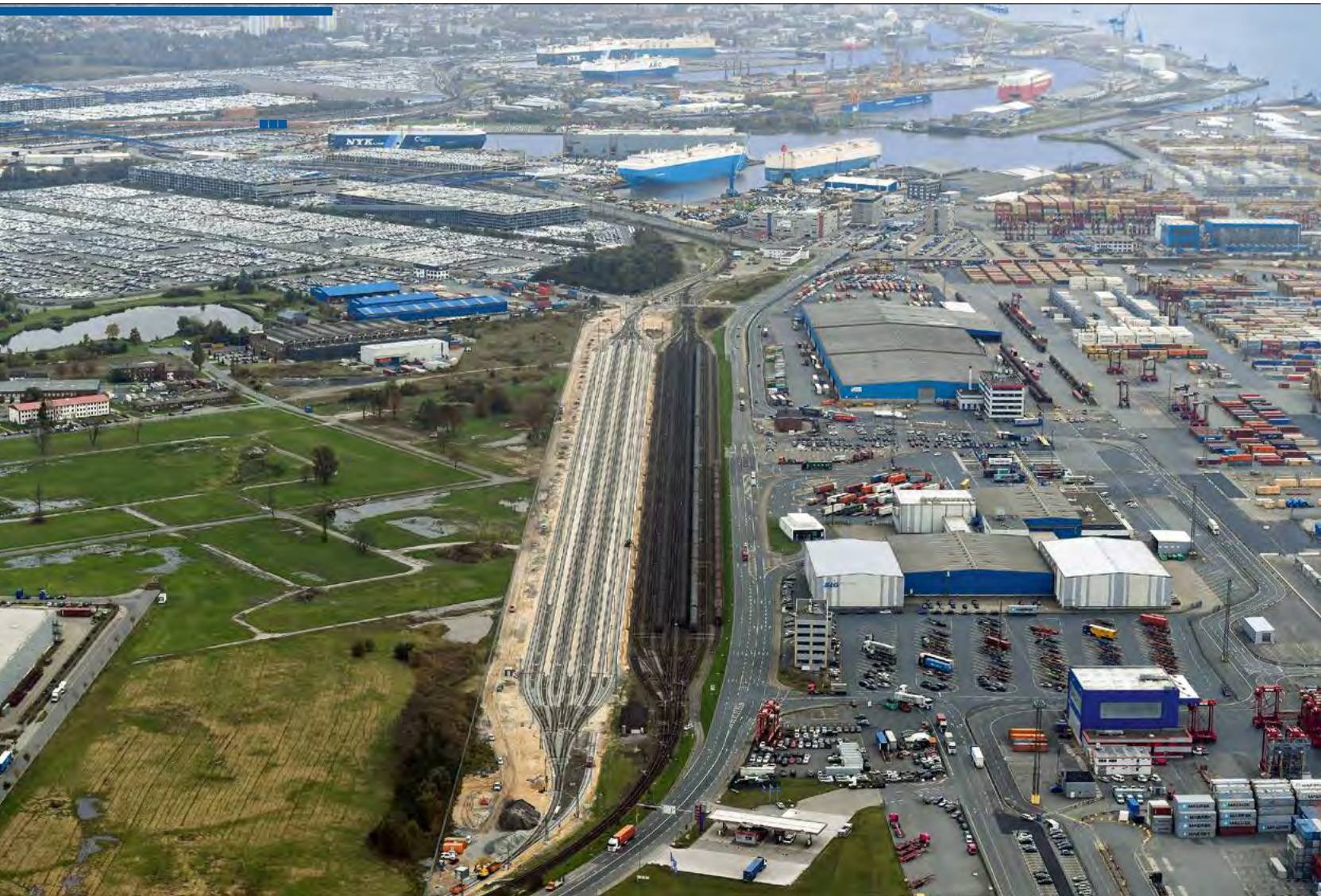
Aerial image of the new tracks at Imsumer Deich in Bremerhaven.
