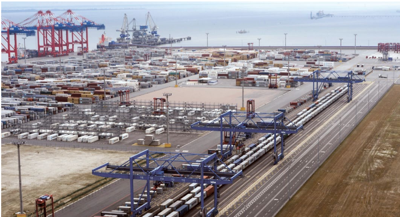
A modern handling terminal with access for deep ships: three gantry cranes on the six 700 metre-long tracks take care of loading sea containers onto trains.
