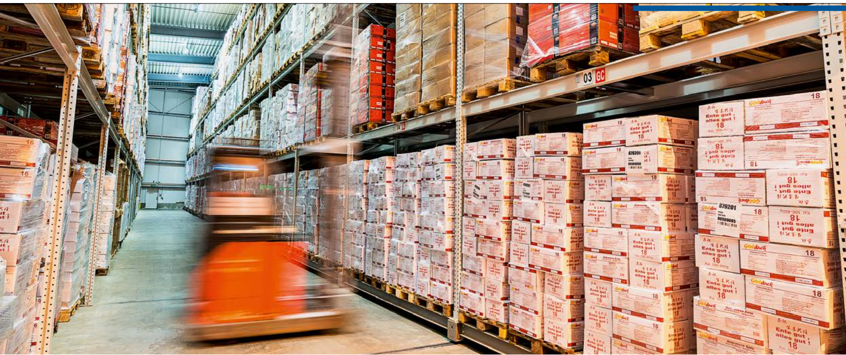
Kloosterboer BLG Coldstore stores frozen and chilled raw materials for the food industry over an area of more than 36,000 square metres.
