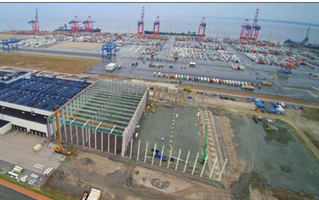
By the start of 2018, the seaport terminal in Wilhelmshaven will be expanded at a cost of 25 million euros.
